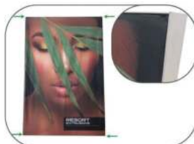
Begin inserting SEG beading at each corner.
